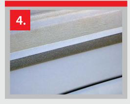
4. Ensure that the paintwork is dry before de-masking.
